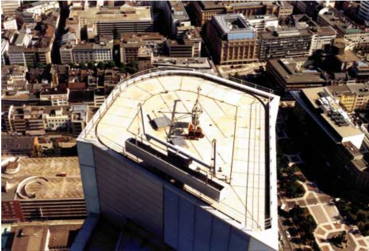
View from Commerzbank to Commerzbank Tower 1 (260m)
