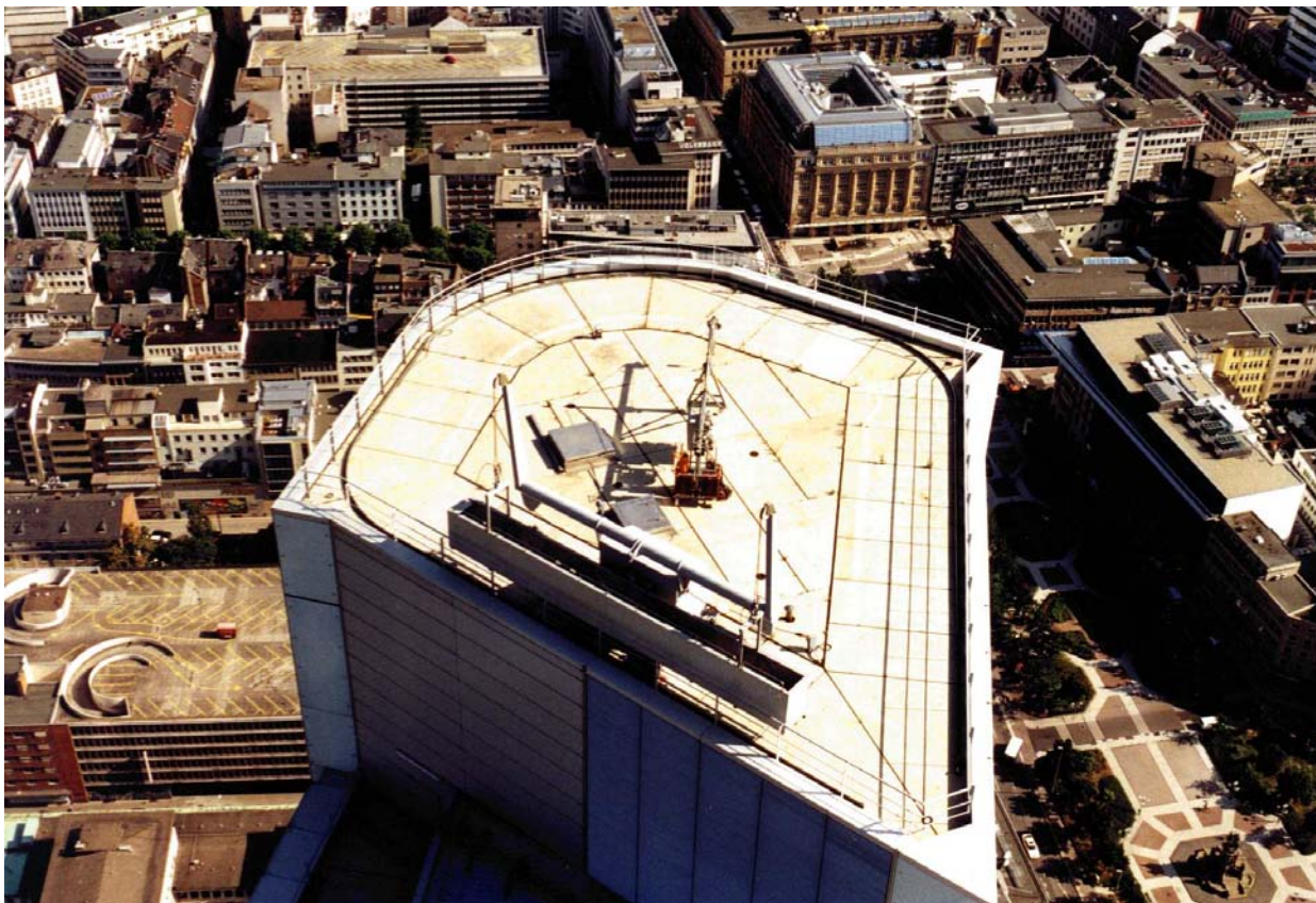
View from Commerzbank to Commerzbank Tower 1 (260m)
